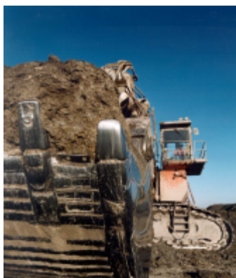
Figure 10 - Excavator at work on an opencast coal mine
