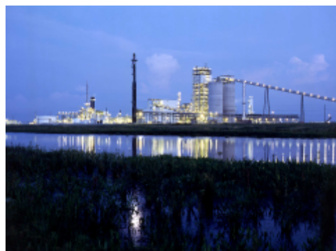
Figure 12 - A modern coal gasification power station (courtesy of Chevron Texaco)
