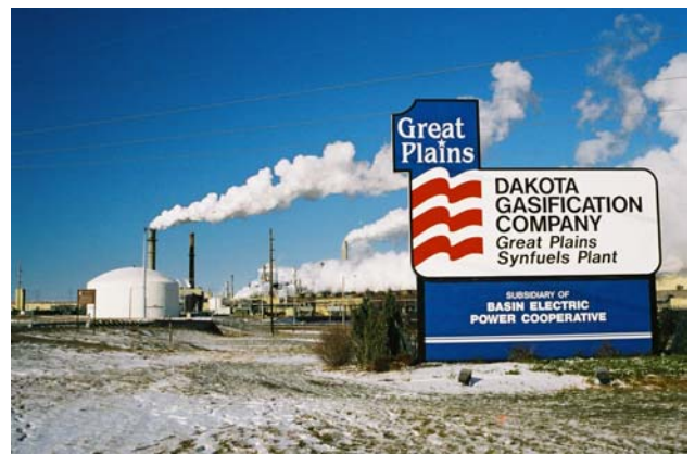
Figure 13 – Dakota Gasification Company’s Great Plains Synfuels Plant at Beulah, USA converts low grade coal into high quality gas that is piped to domestic and industrial users – carbon dioxide (CO 2 ) is captured at a commercial-scale using the Rectisol process (physical absorption by a non-reacting methanol solvent) at this plant for export to Canada
