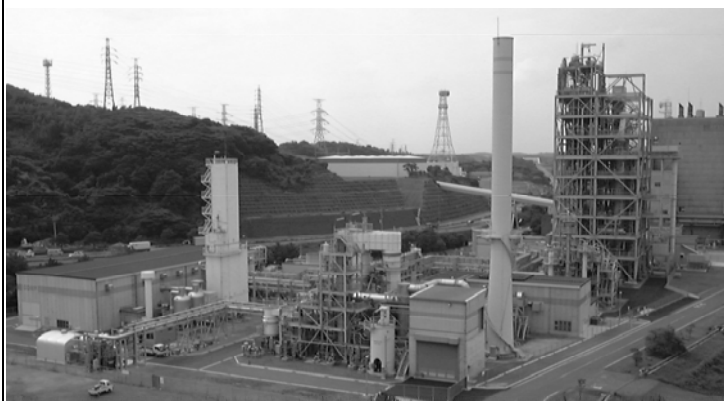
Figure 15 – Japan’s EAGLE project will demonstrate how electricity can be generated using clean and efficient fuel cells fed with hydrogen produced from coal in an integrated gasification combined cycle (IGCC) plant
